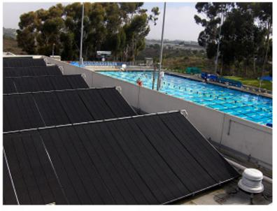
SOLAR THERMAL SYSTEM USED TO HEAT WATER TO 85 DEGREES.
